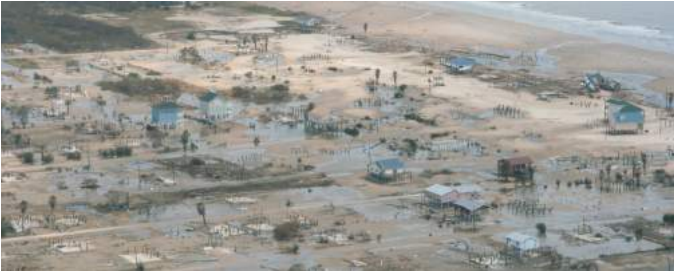
■ FIGURE 6.15 Extensive destruction and damage to a community along the Texas Gulf Coast caused by the storm surge generated by Hurricane Ike in 2008.
