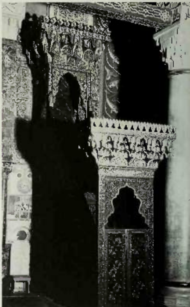
222. Wood screen in Great Mosque, Jerusalem (now destroyed). Dated between 1168 and 1174
