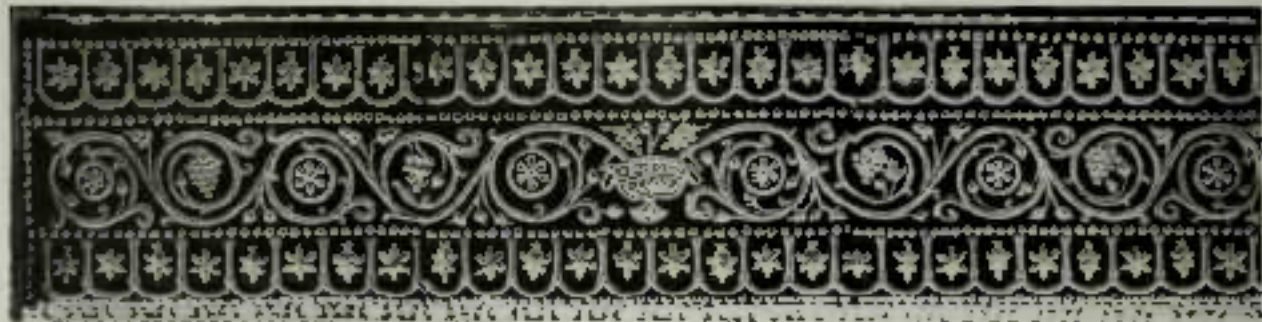
55. Stone frieze, beams covering the Dome of the Rock, Jerusalem, completed c. 691.
