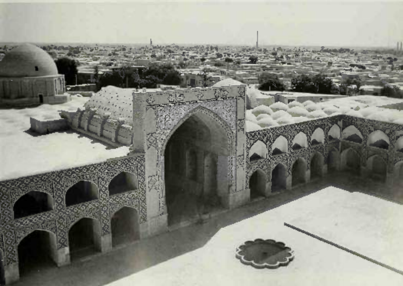
212. Nizamiyya, Mosque, court, Ak-mihrab (left) and the mihrab (right).
