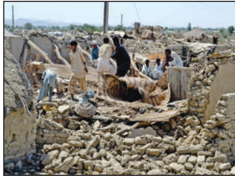
Destruction by earthquakes
