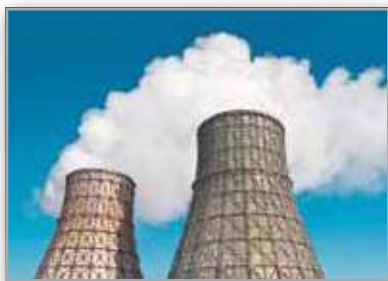
Nuclear cooling towers such as those shown above are in the shapes of hyperboloids. The vertical cross sections of these cooling towers are hyperbolas.
