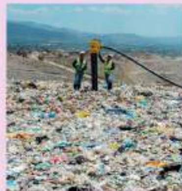
Methane is extracted at the Payatas landfill, Manila—the first in the Philippines to have the gas converted to energy, as part of a United Nations program.
