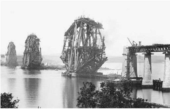
8. The Forth Bridge under construction, 1888-9, completing the railway network, which reached its zenith in the 1890s
