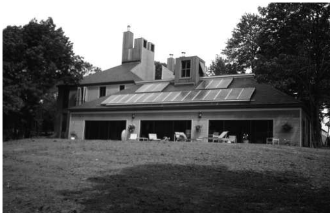
Fig. 28. Solar heating for a pool house. Private Residence, CT. Architect: Charles W. Moore, FAIA. Solar design and engineering: Everett M. Barber, Jr. 1973.
