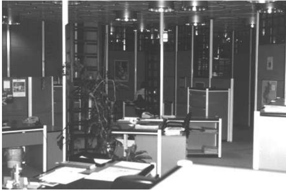
Fig. 9. Modular reconfigurable ceiling with plug-in capability to add or subtract fixtures with various workstation layouts. Colonia Headquarters, Cologne, Germany (ABSIC).
