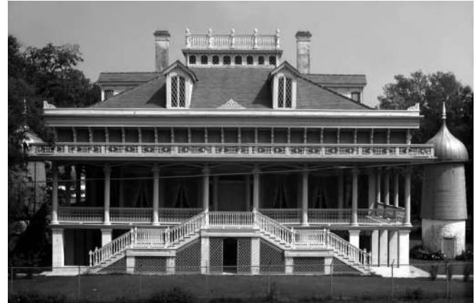
Fig. 17. "San Francisco" a restored manor near New Orleans. Shading and ventilative cooling provided by porches, cross-ventilation, and double-roof "thermal chimney" construction. Photo: Robert Perron.
