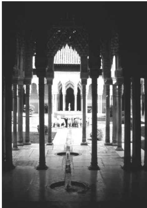
Fig. 18. Palace of the Alhambra, Granada, Spain. 14th Century. Combination of shading, thermal mass and evaporative cooling create a comfortable microclimate. Photo: Cesar Pelli.
