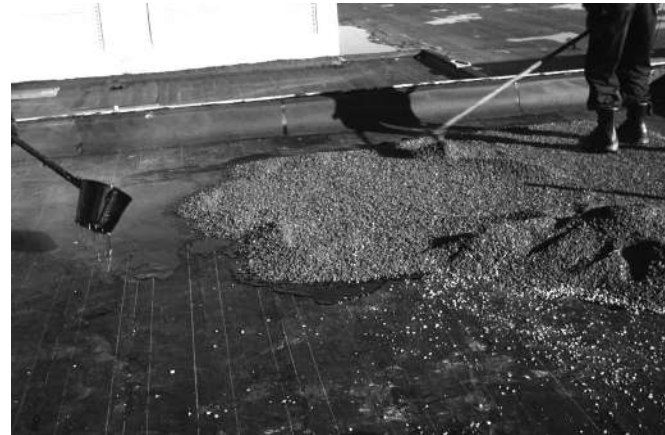
Fig. 2. Pouring asphalt over built-up roof felts, and embedding gravel aggregate.
