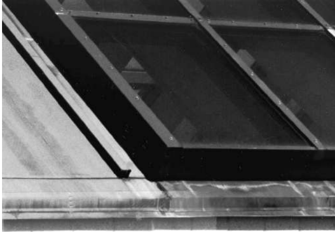
Fig. 13. Copper roof with well-developed light green patina. Below the glass and aluminum skylight, the patina has been removed by acid runoff.
