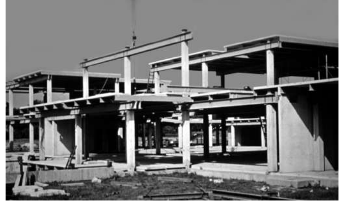
Fig. 7. Free University of Berlin. Demountable concrete and steel panel construction. Shadrach Woods of Candilis, Josic, Woods, Architects.
