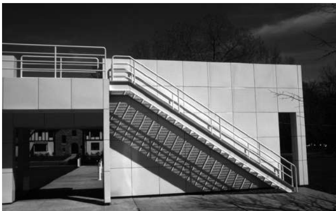
Fig. 6. Hartford Seminary. Ironwork and enamel panel construction. West Hartford, CT. Richard Meier, Architect.
