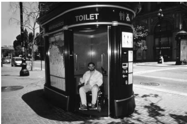
Fig. 8. Public toilet accommodating all users including families. Automatic sensor controls of plumbing. Visual and tactile operating instructions in various languages. San Francisco, CA. J. C. Decaux International with Ron Mace and Barry Atwood.
