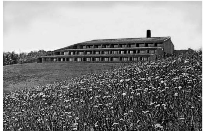
Fig. 15. Scantion Student Housing near Aarhus, Denmark. Earth-sheltering and solar design. K. Friis and E. Moltke, Architects.
