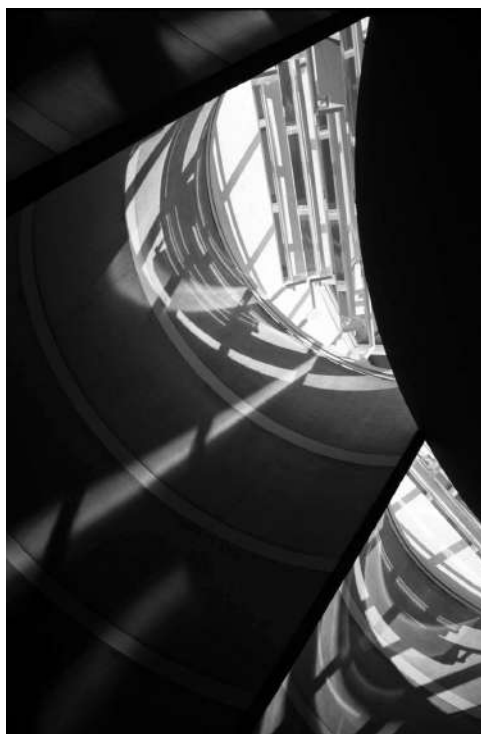
Fig. 11. Skylights of the Chapel at Harvard Business School, Cambridge, MA. Architect: Moshe Safdie; Sculptor: Charles Ross; Prism steering design and installation: Thomas Hopper. 1990. Oil-filled prisms are computer-controlled to track the sun and create a continuously refracted sunbeam.
