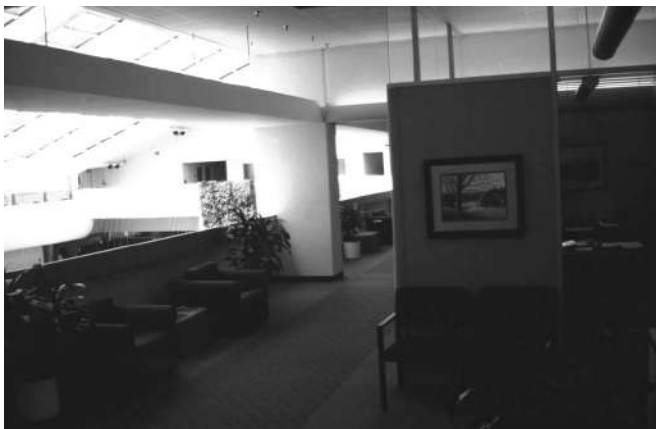
Fig. 4. Light reflectors along the interior of TVA Headquarters atrium
