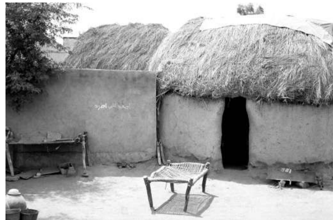
Fig. 13. Adobe home. Al Hudaydah, Yemen. Located in a hot humid area on the Red Sea, most summer hours are above the comfort zone. The sleeping cot in the courtyard provides some relief and radiant/ventilative cooling comfort at nighttime.
