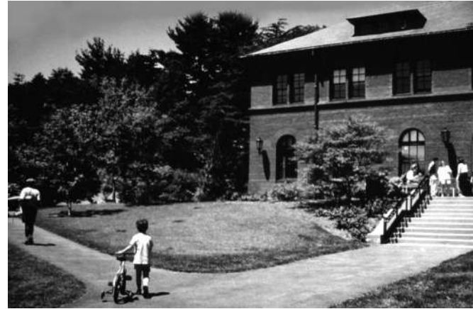
Fig. 4. Renovated entry landscape with sloping walkway and outdoor seating platform to Hunnewell Visitors Center at the Arnold Arboretum, Jamaica Plain, MA. Carol R. Johnson Associates, Landscape Architects.
