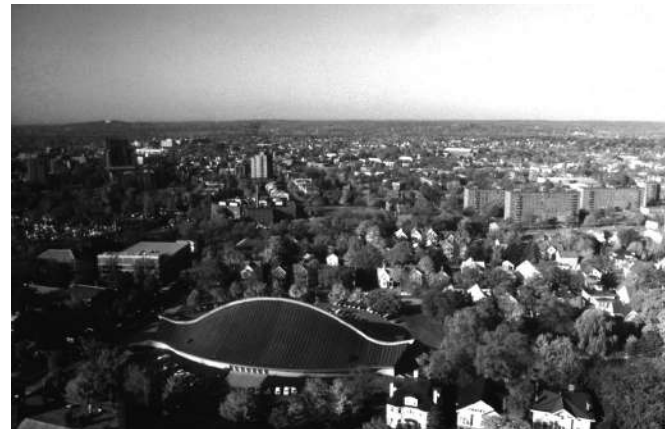
Fig. 3. Thermoset membrane roof, Ingalls Ice Skating Rink, Yale University, New Haven, CT. Eero Saarinen, Architect; F. J. Dahill Co., Roofing Contractor. The membrane roof protects surfaces that vary from very steep to low slope and accommodates flexing of the structure. 1957.
