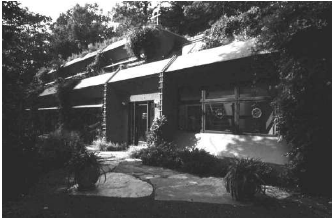
Fig. 14. Earth-covered Home. New Canaan, CT. Earth-sheltering and solar design. Donald Watson, FAIA, Architect and Builder.
