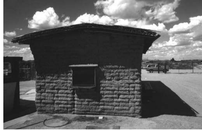
Fig. 12. Adobe home. Papago Indian Nation, Arizona. A centuries-old building tradition evident in informal house construction provides thermal time delay in hot-arid climate. Overhangs provide shading and protect the adobe
