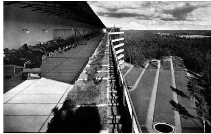
Tuberculosis Sanatorium. Paimio, Finland. Alvar Aalto, Architect. 1928-33.
