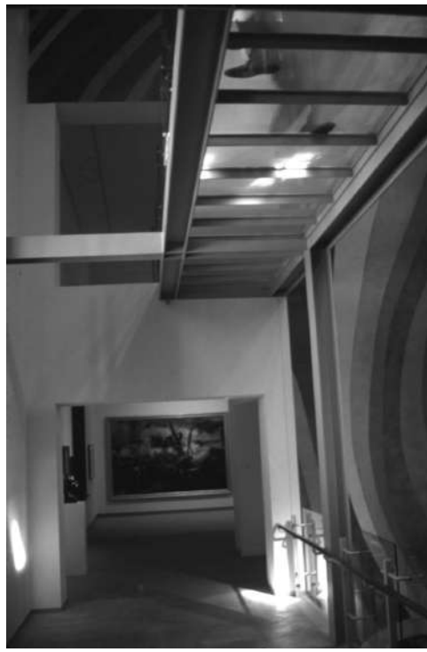
Fig. 12. Atheneum Museum, Hartford, CT. Remodeling of Entryway. 1996. Glass walkways (seen above at right of photo) diffuse daylight throughout the entry gallery. Ta-Soo Kim, Architect.
