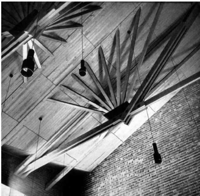
Fig. 4. Expression of structural truss. Saynatsalo Town Hall.
