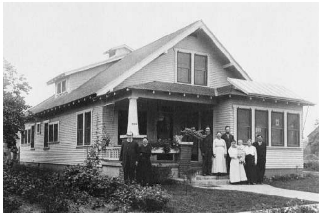
Fig. 4. The "Day and Night" solar water heater, so named because the addition of an insulated "thermosyphon" tank inside the dwelling attic provided stored solar heated water for use at night. Seen here in a Pomona Valley, CA installation circa 1911. (Butti and Perlin 1980).
