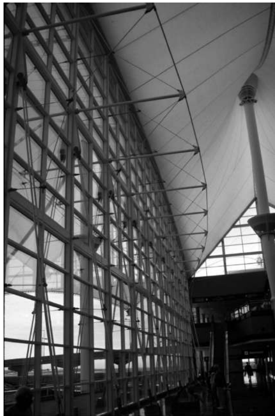
Fig. 5. South wall of Denver International Airport Terminal.
