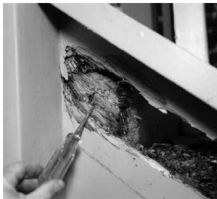
Fig. 4. Termite damage
