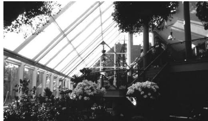
New Canaan Nature Center Solar Wintergarden, New Canaan, CT Buchanan/Watson Architects 1984
