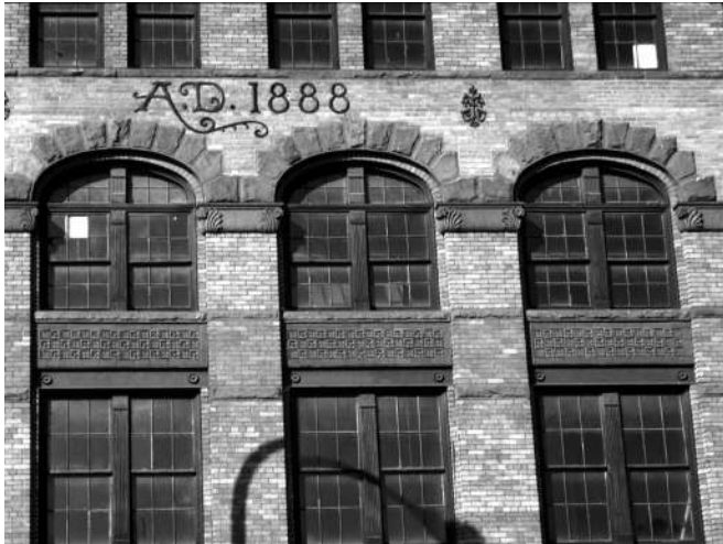
Fig. 1. Brick wall construction with terra cotta tilework. Troy, NY.
