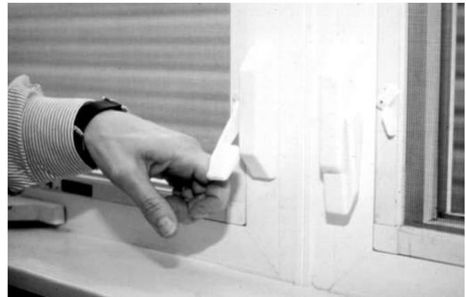
Fig. 15. Window Lock/Latch, accommodating dexterity limitations and “aging in place.” Owens Residence, Chicago, IL. Design One, Industrial Design.
