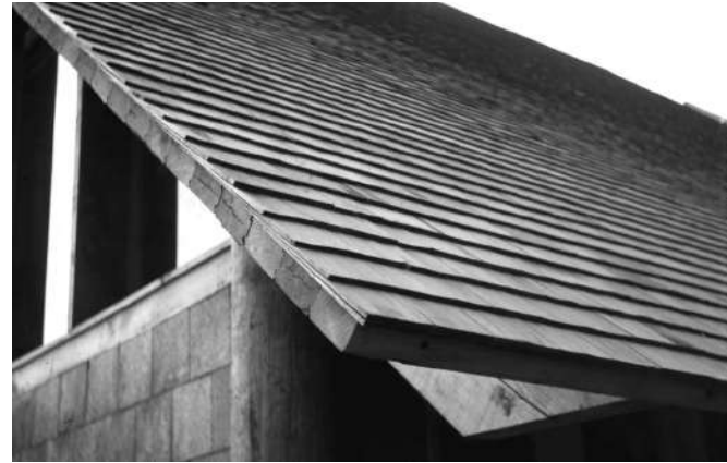
Fig. 11. Western redcedar shingle roof on First Presbyterian Church, New Haven, CT. John Dinkeloo, Architect. 1966.
