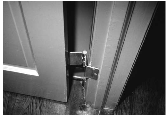
Fig. 14. Swing Clear Hinge, allowing a door to be fully opened for wider access. Gilreath and Associates, Interior Designers.
