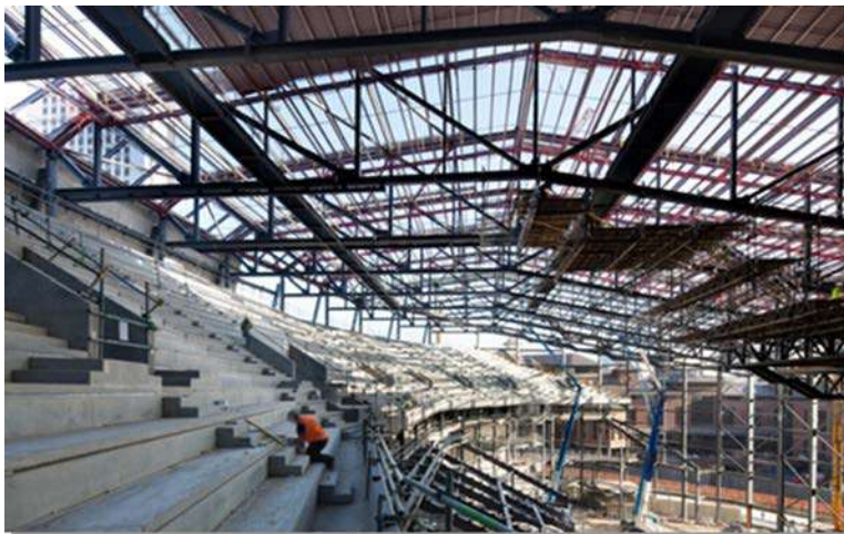
Arena during construction.
