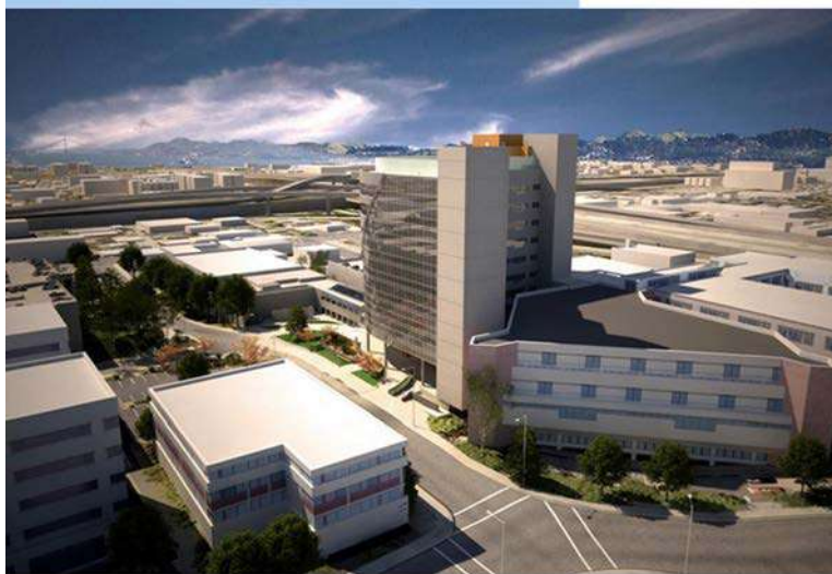
PCP tower adjacent to the existing hospital.
