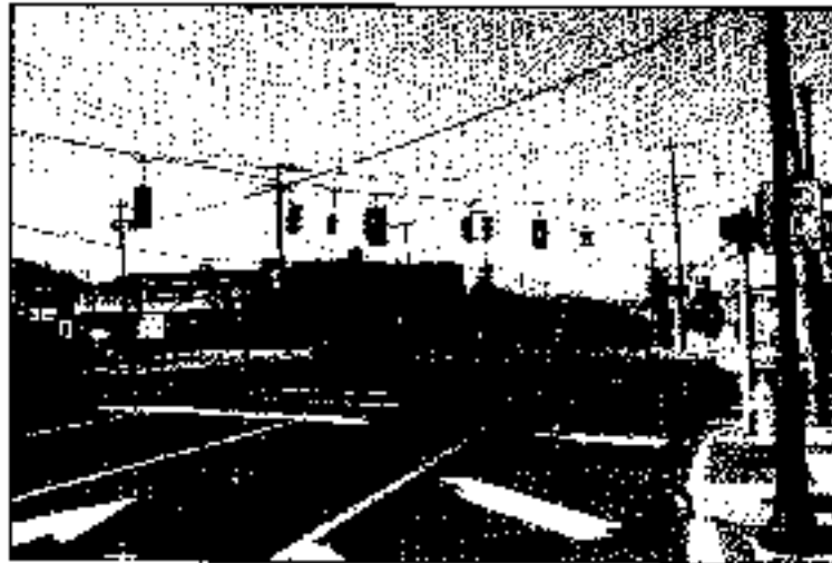
Figure 19.30: A Typical Span-Wire Signal Installation
