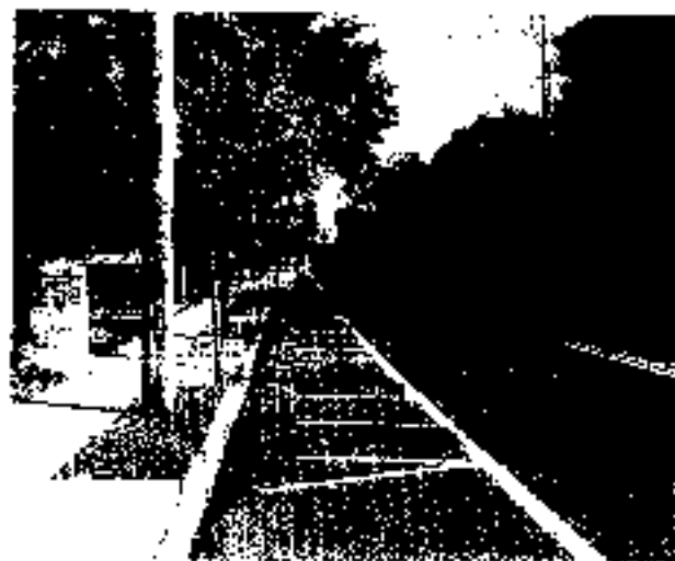
Figure 3.21: Sight Distance Limited by a Crest Vertical Curve
