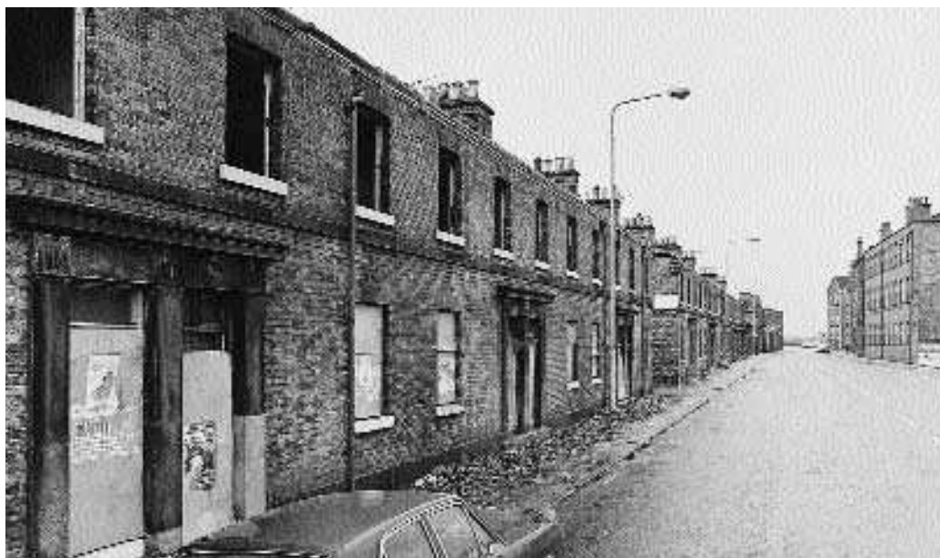
Figure 5.22 Railway Cottages, Derby. Before rehabilitation.
