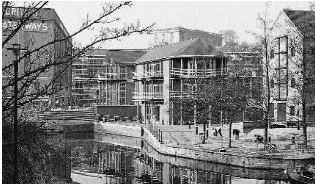
Figure 4.17 Canalside development, Nottingham: offices and restaurants.
