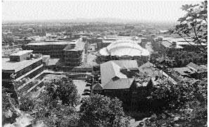
Figure 4.13 Canalside development, Nottingham: The Inland Revenue Building by Michael Hopkins and Partners.
