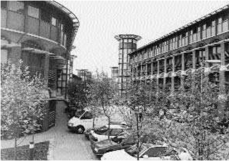
Figure 4.14 Canalside development, Nottingham: The Inland Revenue Building by Michael Hopkins and Partners.
