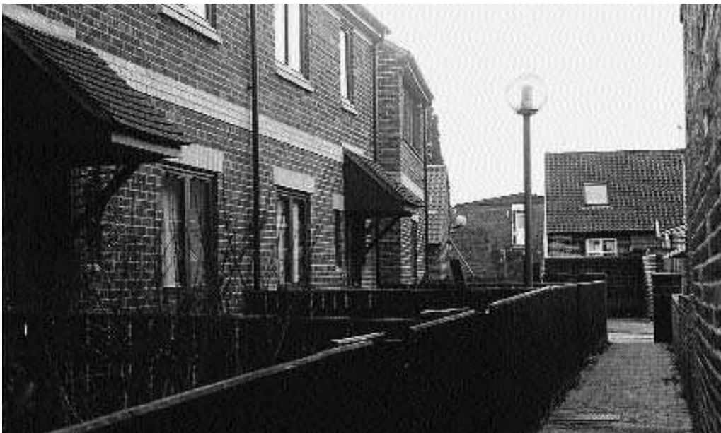
Figure 5.48 Millgate. Completed project.
