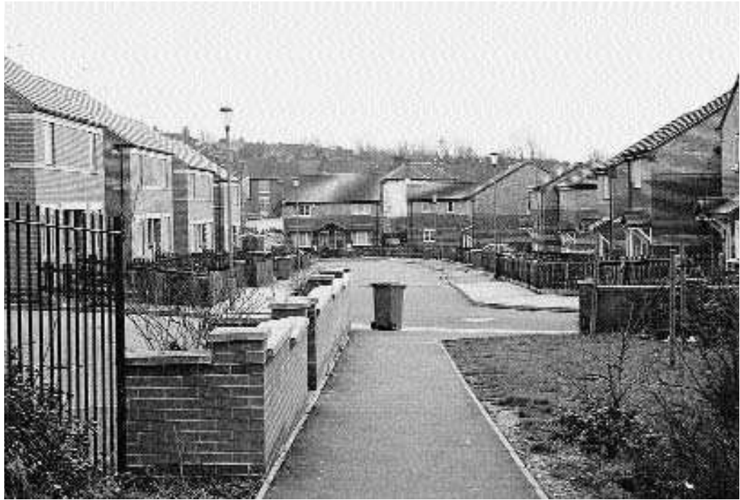
Figure 3.1 Radford. A return to a street architecture after demolition of 1960s deck access flats.
