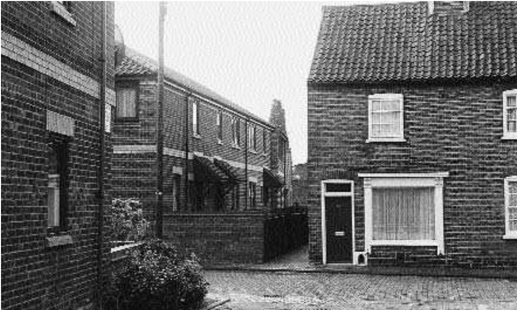
Figure 5.47 Millgate. Completed project.
