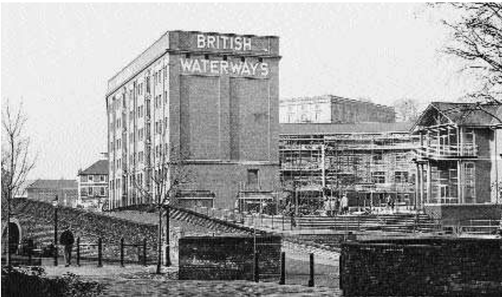
Figure 4.16 Canalside development, Nottingham: refurbished warehouse.
