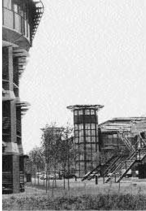
Figure 4.12 Canalside development, Nottingham: The Inland Revenue Building by Michael Hopkins and Partners.
