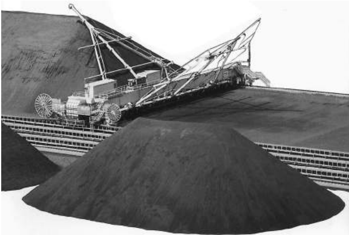
FIG. 21-48 Recovery of the fine homogenized coal by system Chevron (Central Coking Plant, Saar GmbH, Germany); width of the bridge scraper is 57.5 m; capacity is 1200 t/h. (Courtesy of PWH-Krupp Engineering.)
