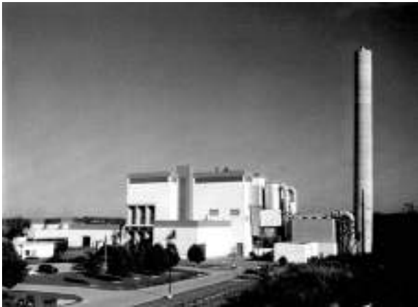
FIG. 22-52 1200-tons/day MSW plant of Montenay Montgomery.
