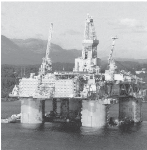
Figure 12 Demands of the superstructures of offshore oil rigs in high humidity and water exposure are met with 5454, 5086, and 5083 Al–Mg alloy welded construction. (Courtesy of the Aluminum Association.)
